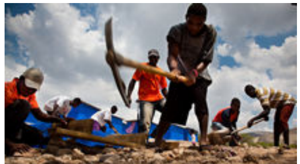
Clearing ground for shelter in Haiti
